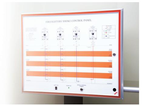
Our meticulously engineered and manufactured panels are tailor made for your project to provide first responders with a consistent, recognizable, code-compliant Firefighter Smoke Control Station (FSCS) ensuring instant manual control and override authority of mechanical smoke control systems.
